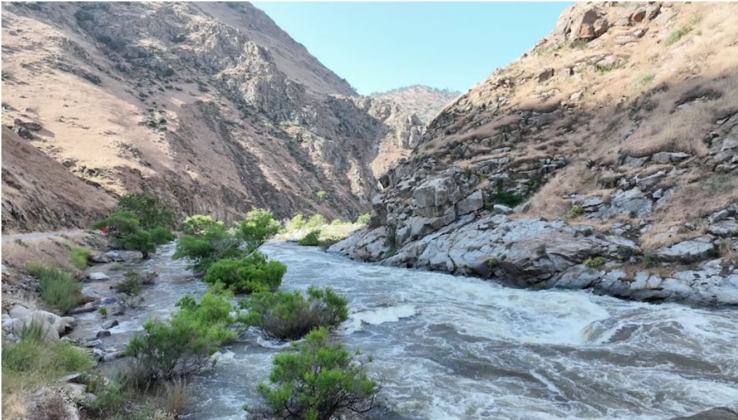
Figure 31. Photo of the Kern River below Isabella Dam (USACE photo).
