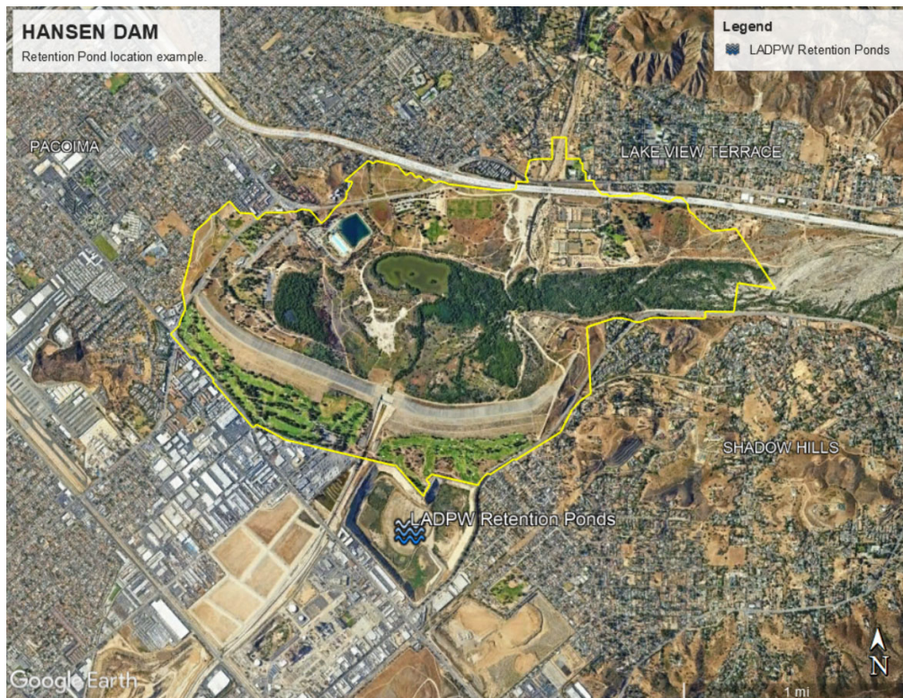
Figure 29. Example of retention pond infrastructure downstream of Hansen Dam.
