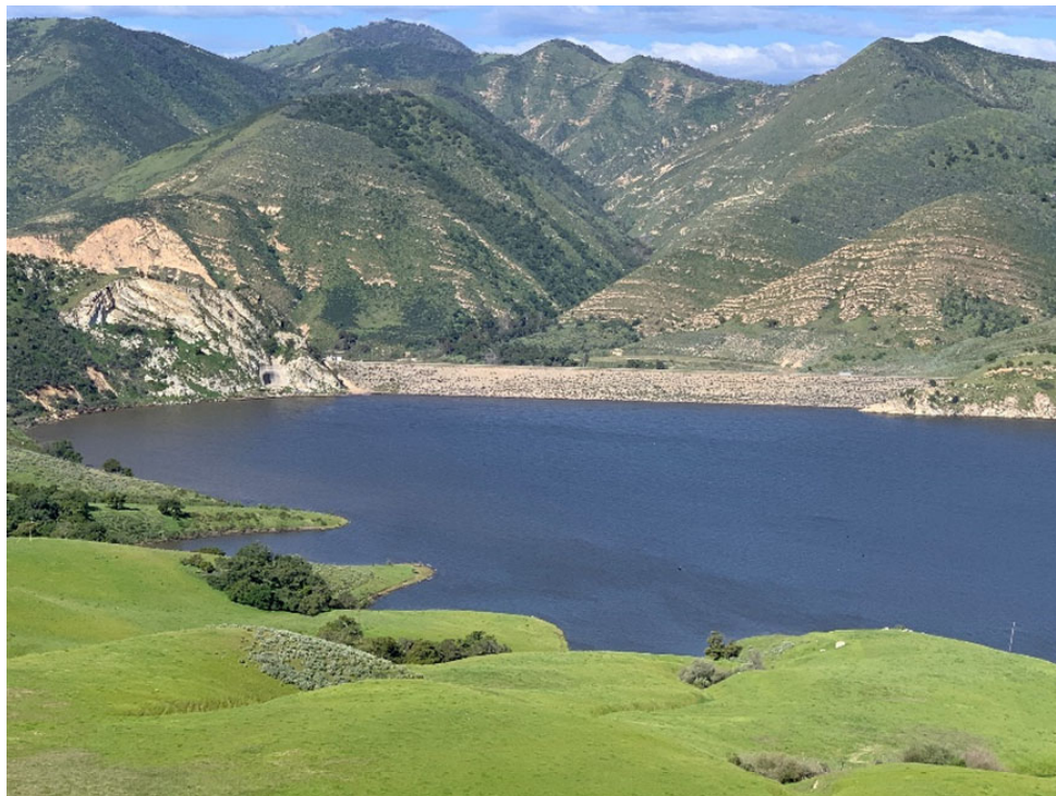
Figure 17. Twitchell Dam and Spillway (USACE photo).
