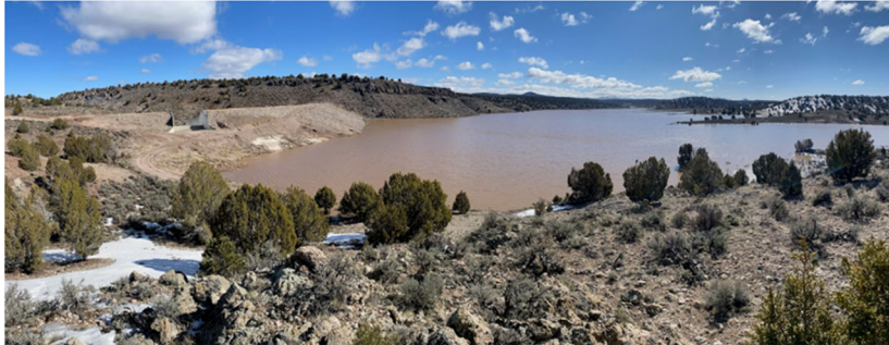
Figure 13. Photos of Mathews Canyon Reservoir and Pine Canyon looking downstream (USACE photos).
